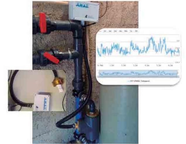
Fig. 2 Water Quality Sensor installed at Segadães (Águeda) water supply network – pipe point oNE. up right: turbidity measurements between 31st MAY and 6th June, 2017.
